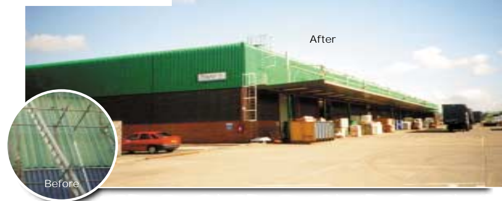
External Walls & Cladding
