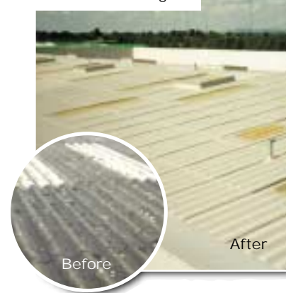
Roofs & Roof Lights
